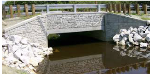
The bridge crossing Dog Creek will accommodate multiple modes of transportation.
