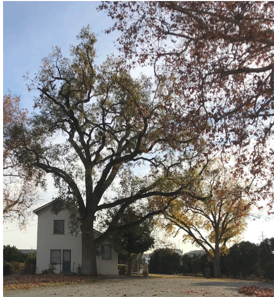
Existing residential structure with stately oak and sycamore trees
